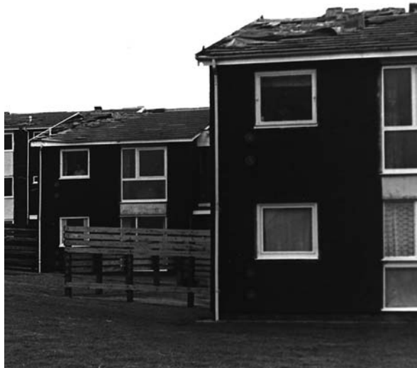
Underlay under negative pressure
